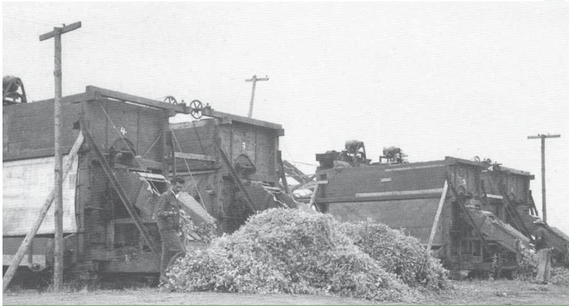
Pea-shelling machines were used in the 1960s to process canned and frozen peas (Friday Harbor).
