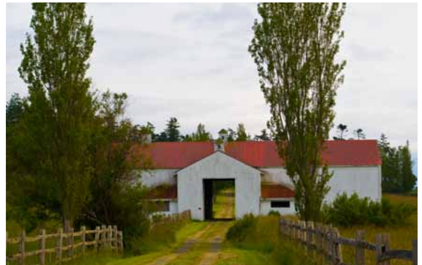
Many unique and colorful, historic barns have been preserved across the islands and are still in use.
